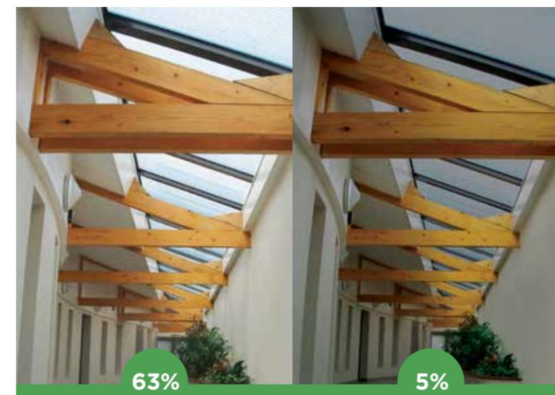
63% of visible daylight is transmitted through Controllite® panels in the OPEN position
